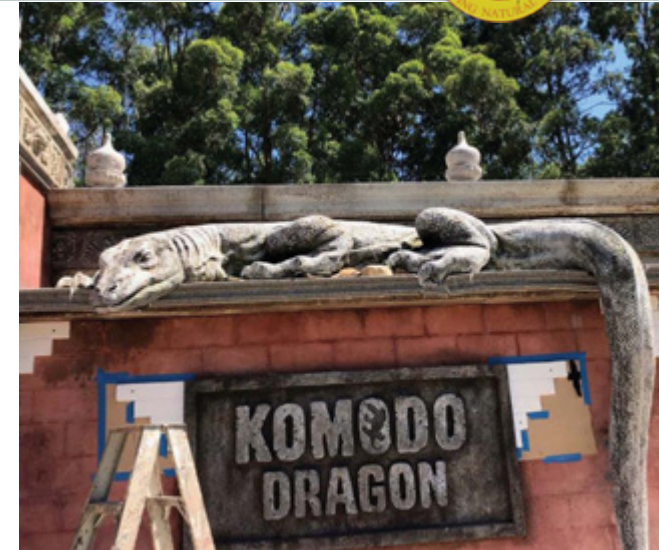
Installing the lizard sculpture
