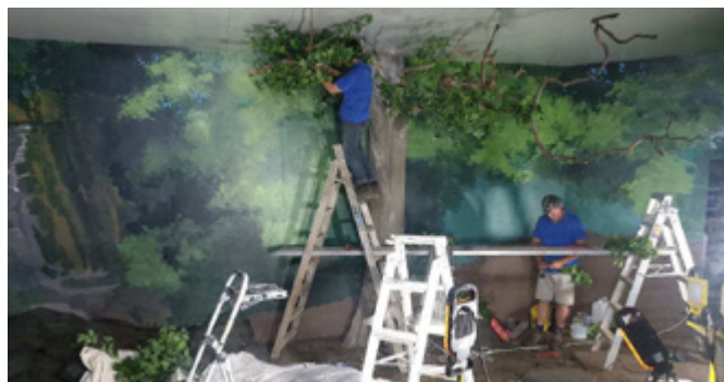
Installing artificial trees
