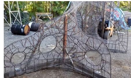
Steel reinforced substructure
