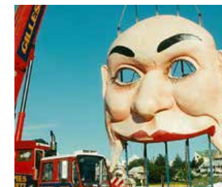
Step 5. Craning the sculpture into position and installing it on site in place of the old sculpture.
